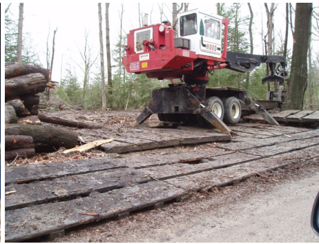
Well Constructed Log Landing
